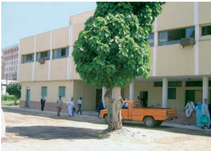
Shebine el Kom, Phase II, Building
